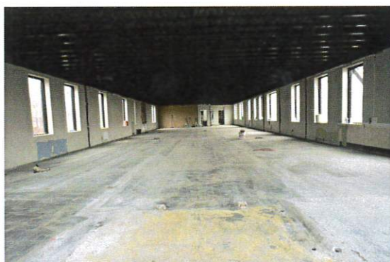
After demo - before renovation
